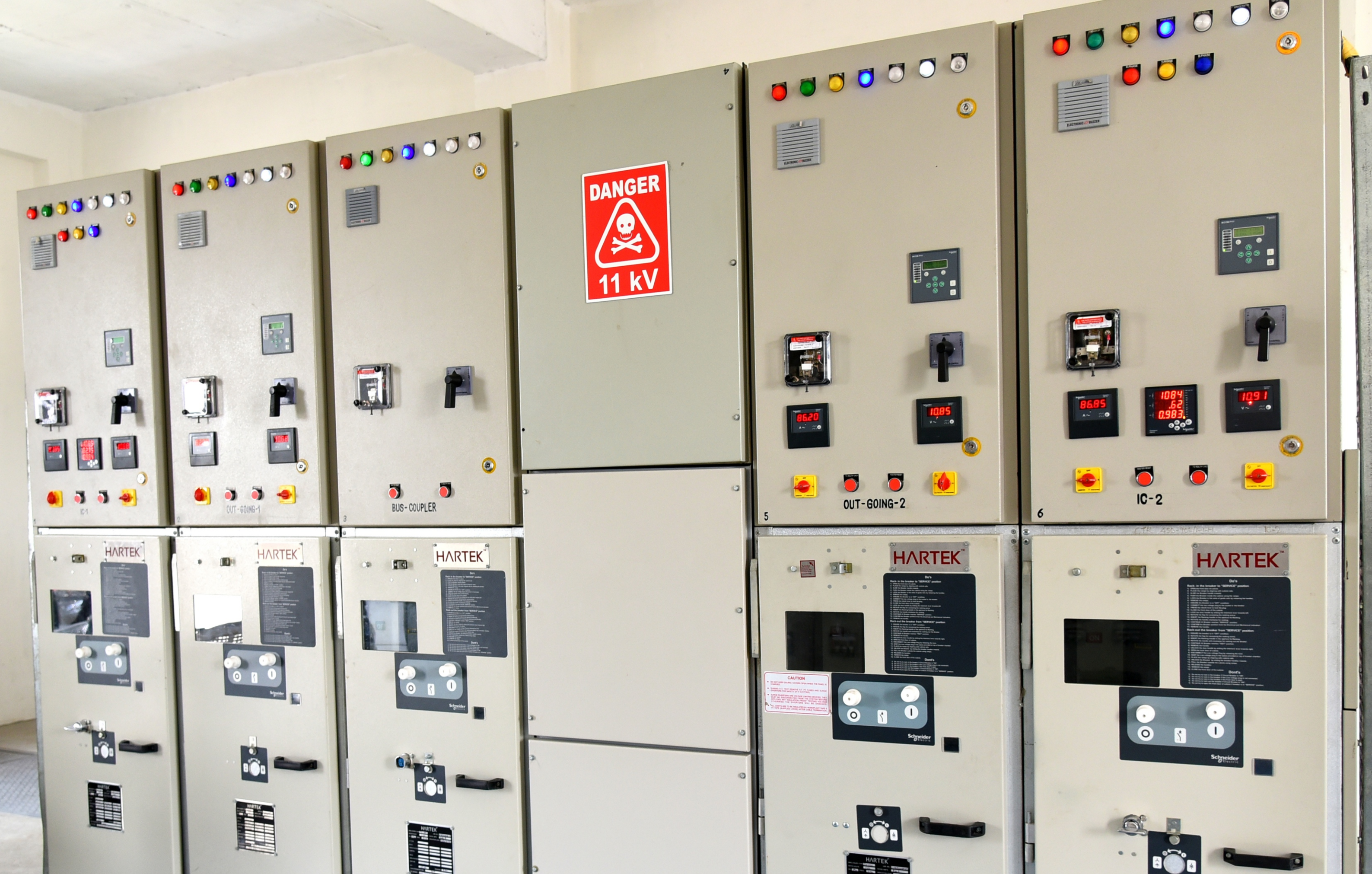
Medium Voltage Switchboard Panel
